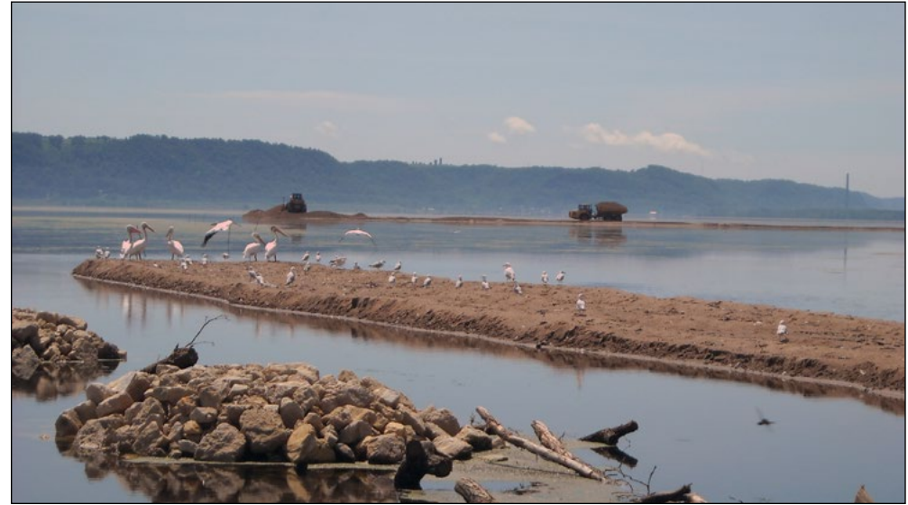
A rock log structure connecting two islands at the Pool 8 Islands project near Brownsville, Wisconsin, June 22, 2010. USACE courtesy photo
